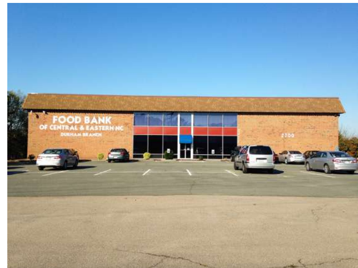
Durham Exchange Club Industries - Food Distribution Center
